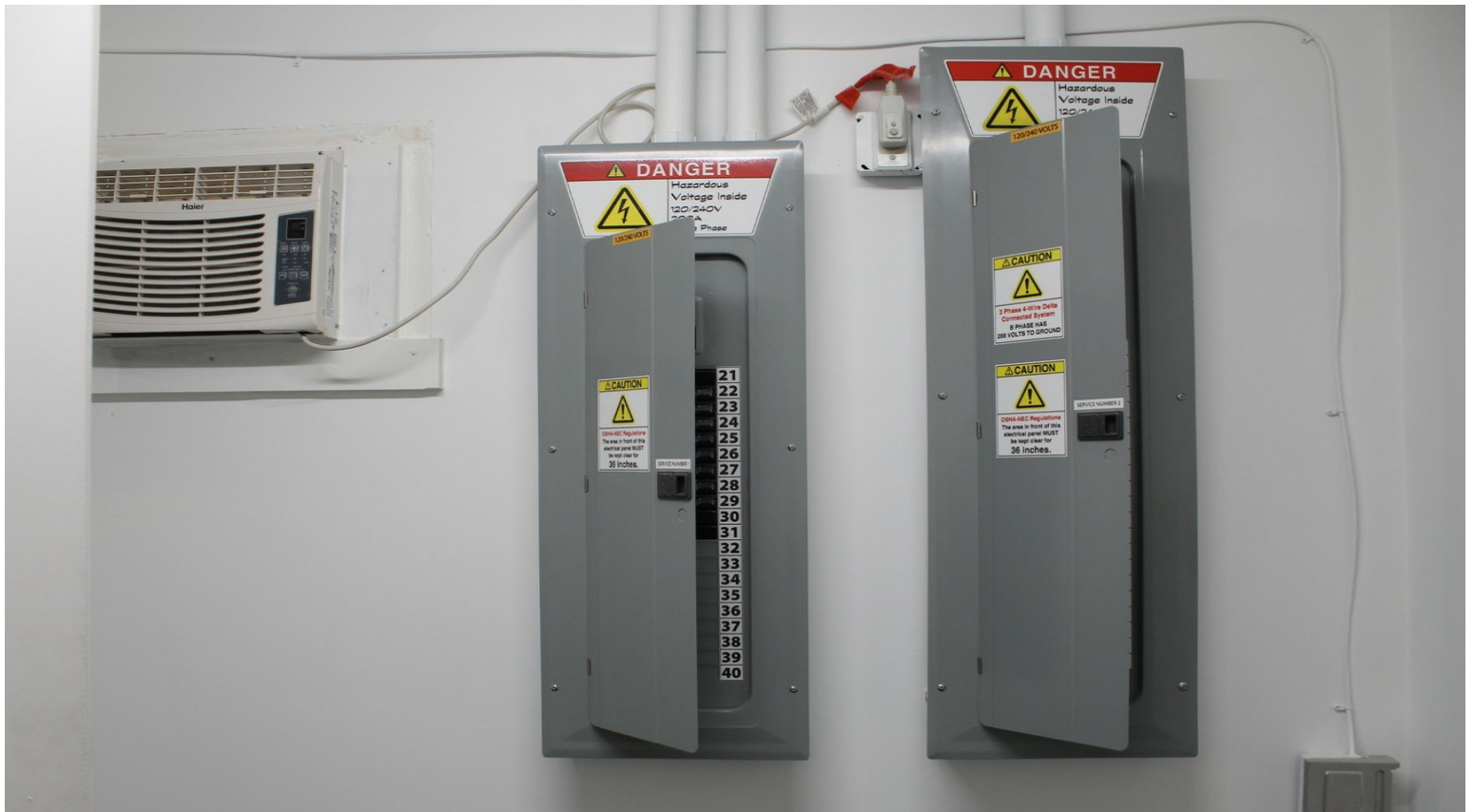
Three Phase, 400 amp Electrical
